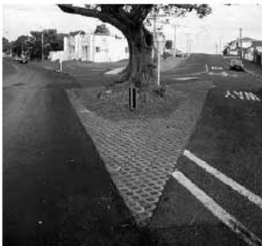
Figure 13. Air for tree roots and a warning for drivers
