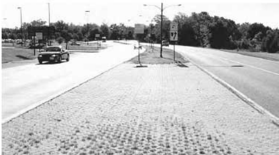
Figure 6. Roadway median crossover
