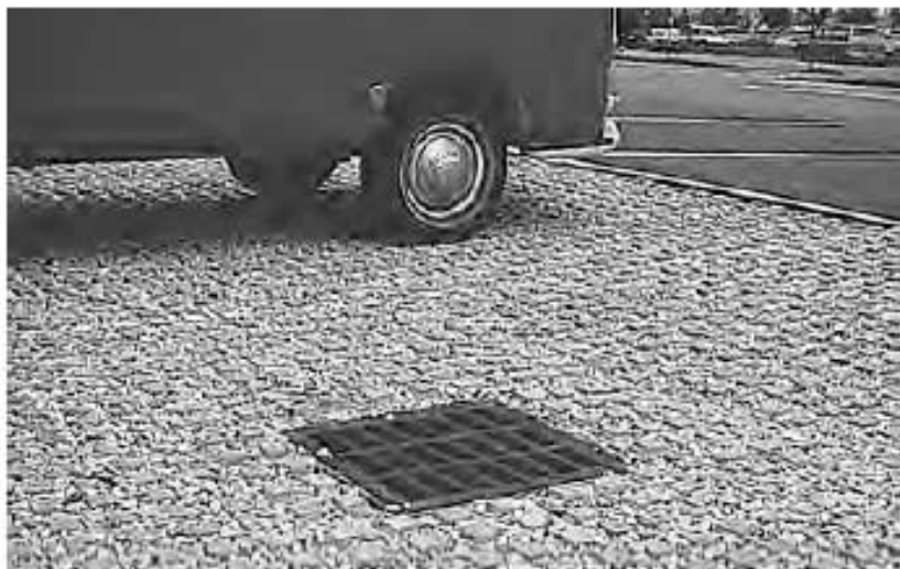
Figure 18. Concrete grids with aggregate in the openings
