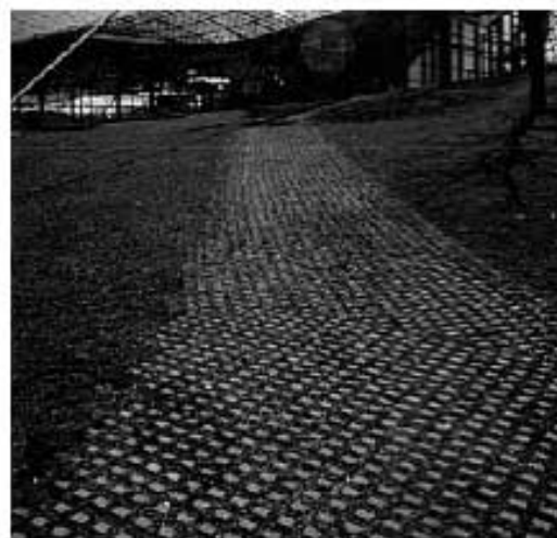
Figure 7. Service access lane
