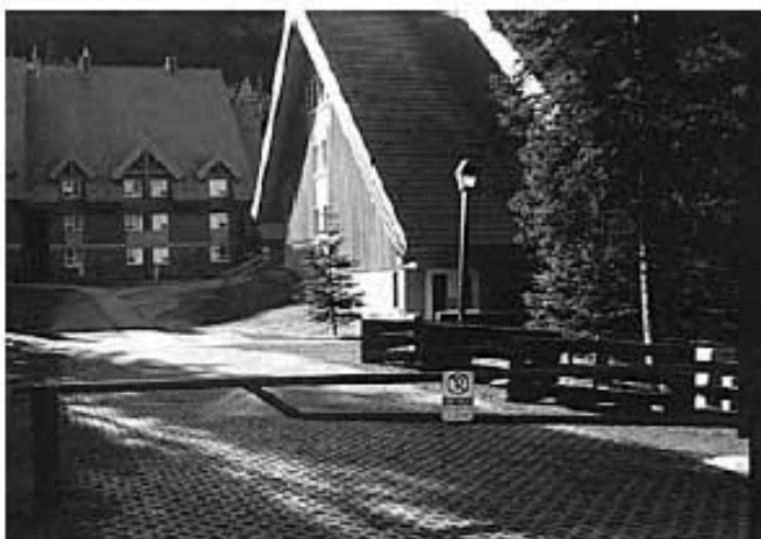
Figure 8. Emergency access lane for fire trucks
