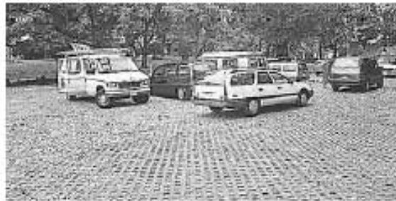
Figure 16. A parking lot with a dense-graded, crushed stone base.
