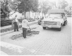
Figure 3. Compaction of the base.
