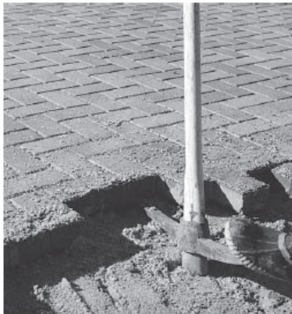
Figure 6. Prying out the remaining pavers
