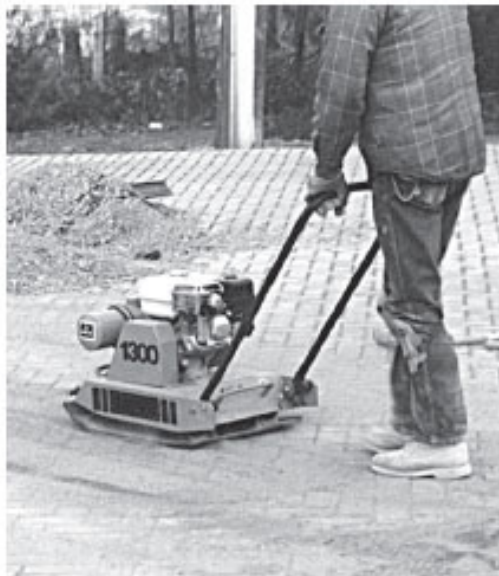
Figure 13 (Left). Adjusting joint spacing and alignment. Figure 14 (Right). Second and final compaction of the pavers. The first compaction occurs after the pavers are placed (no sand in the joints). The second compaction works the sand on pavers into the joints. This process causes the pavers to interlock.
