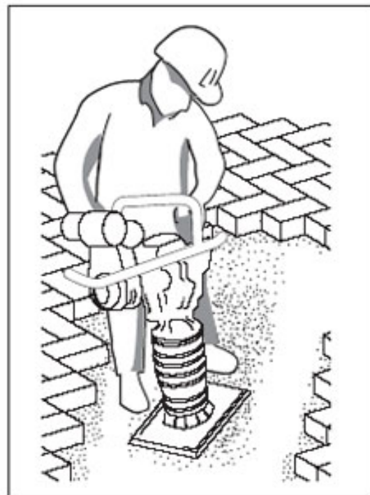
Figure 10. Compaction of the base in 2 to 4 in. (50 to 100 mm) lifts and monitoring density with a dynamic cone penetrometer or a nuclear density gauge are essential to minimizing settlement.
