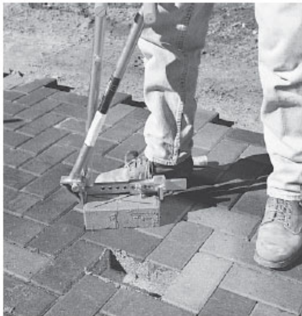
Figure 5. Using a paver extractor to remove a paver
