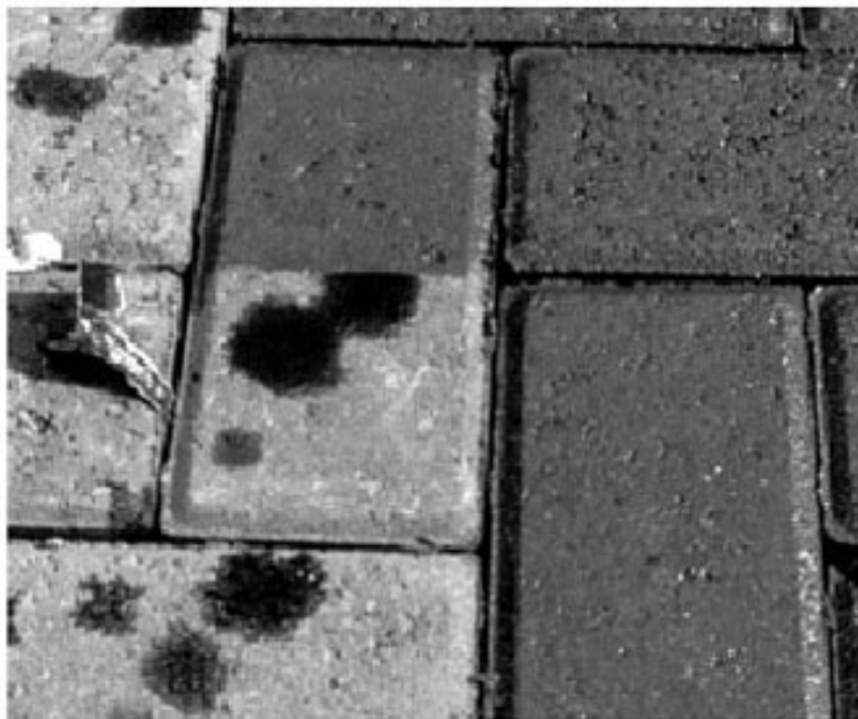
Figure 9. Sealers resist stains which makes them ideal for high use areas where they might occur.
