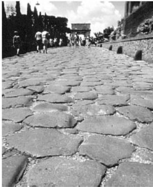
Figure 1. The Roman Appian Way: early interlocking pavement.
