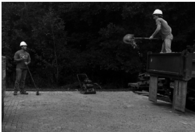
Figure 10. Spreading and sweeping joint sand.
