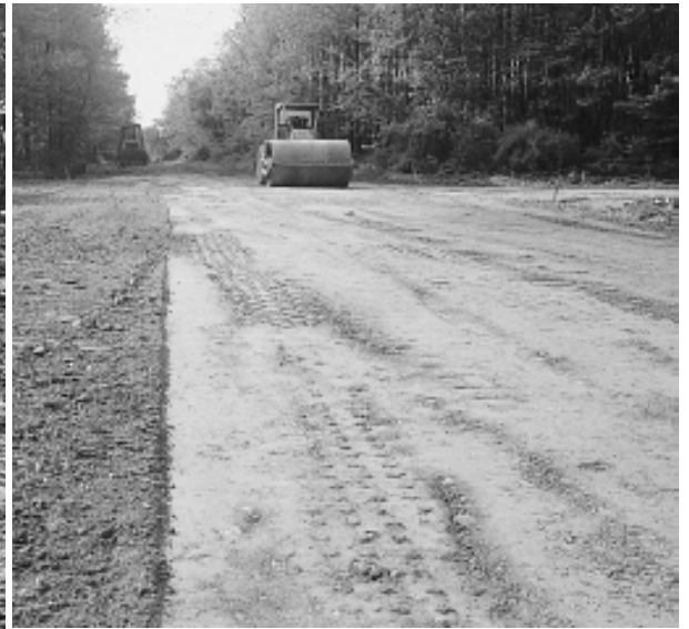
Figure 2. Compacting the soil subgrade.
