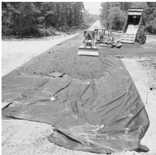
Figure 3. Application of the geotextile under aggregate base.
