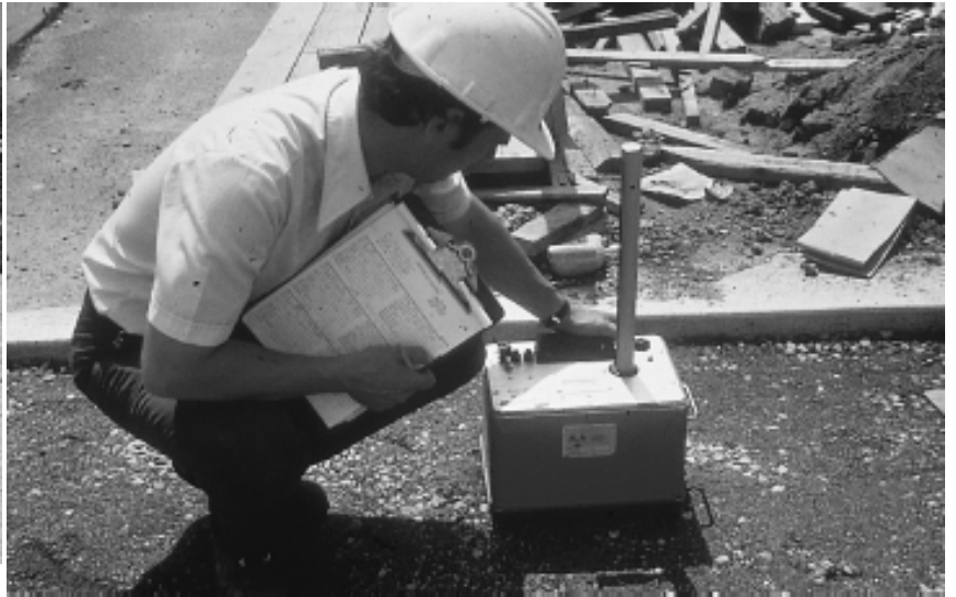
Figure 5. Density testing of the aggregate base with a nuclear density gauge.
