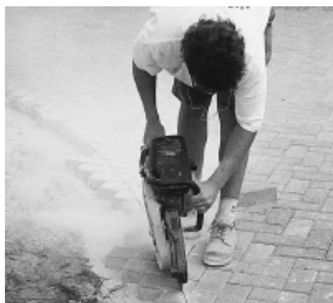
Figure 8. Saw cutting pavers.
