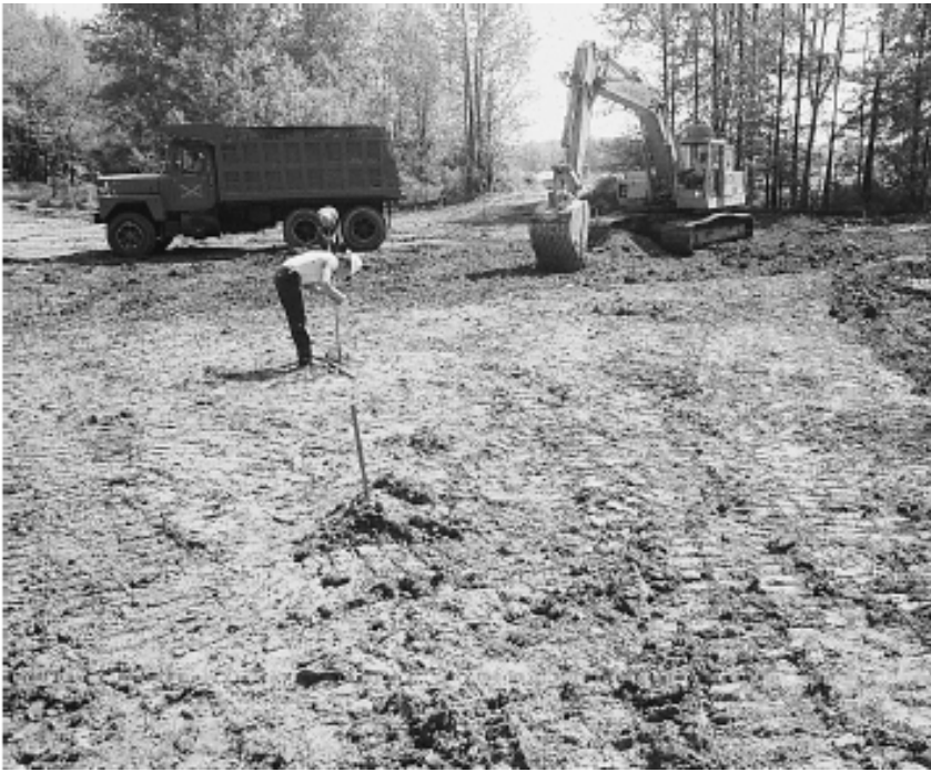
Figure 1. Excavation of the soil subgrade.
