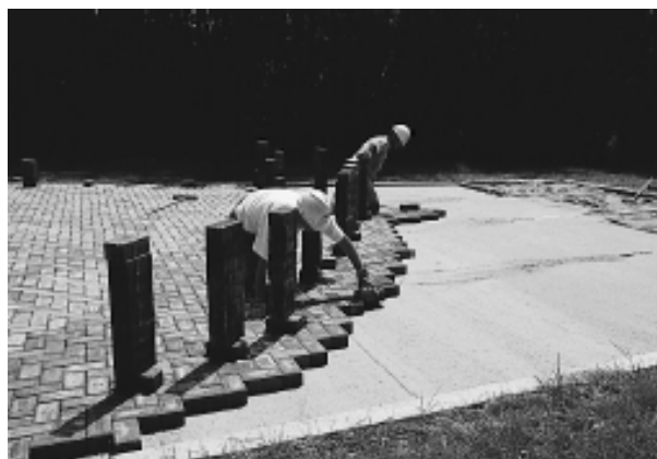
Figure 7. Placing the concrete pavers.
