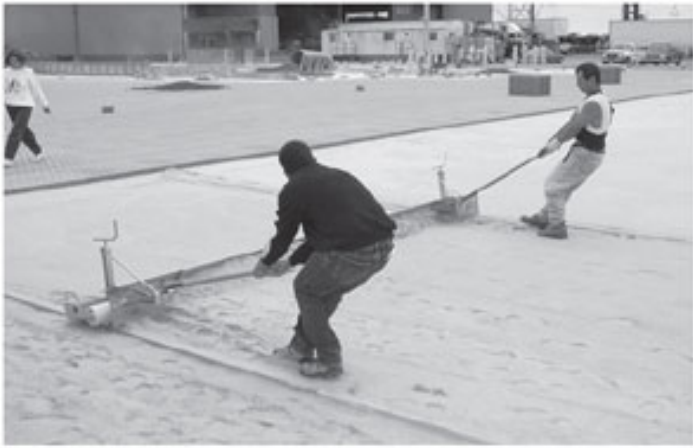
Figure 4. A two-man hand pulled screed
