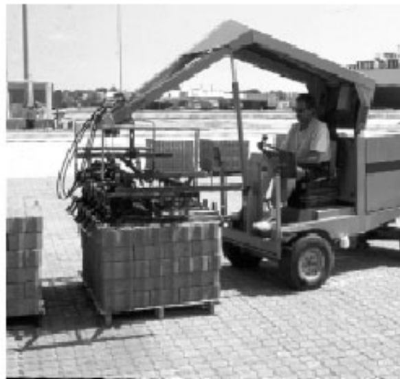
Figure 3. A cluster of pavers (or layer) is grabbed for placement by mechanical installation equipment. The pavers within the cluster are arranged in the final laying pattern as shown under the equipment.
