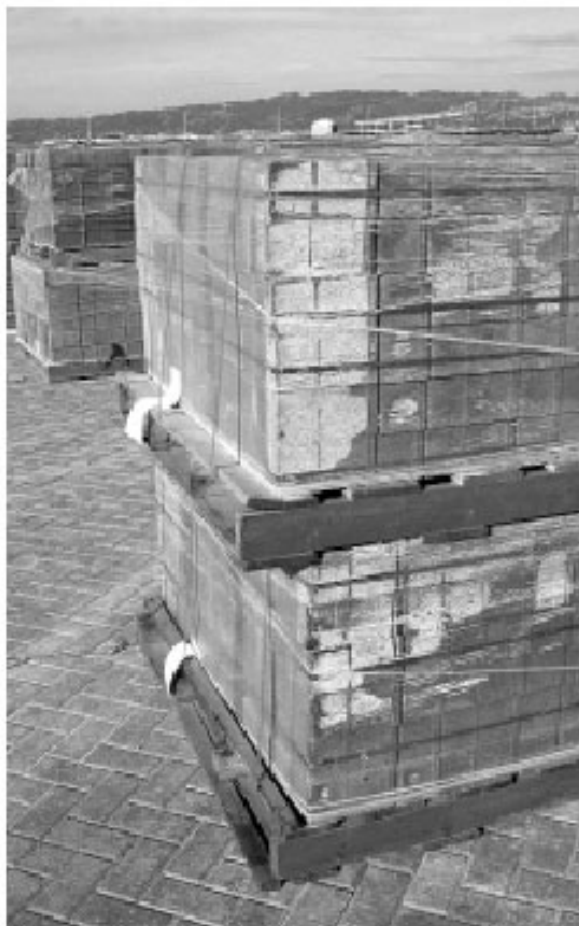
Figure 2. Bundles of ready-to-install pavers for setting by mechanical equipment. Bundles are often called cubes of pavers.
