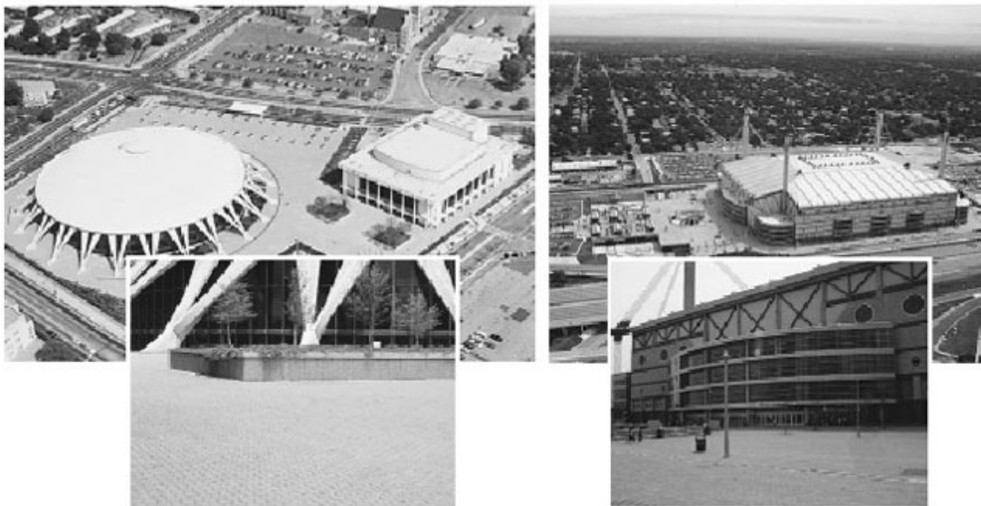
Figure 21. The plaza area around Scope Center in Norfolk, Virginia, (left) and one side of the Alamo Dome (right) in San Antonio, Texas, include roof plaza decks surfaced with concrete pavers.
