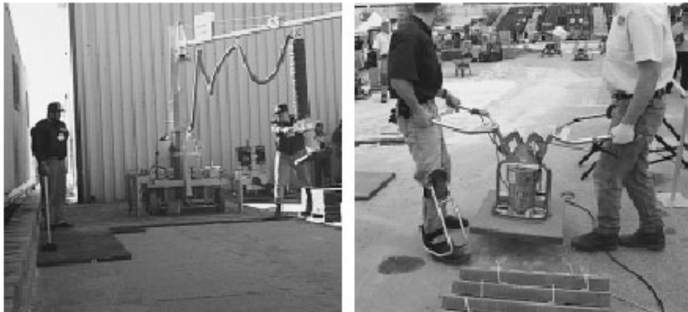
Figure 20. Vacuum assisted mechanical equipment for installing paving slabs.
