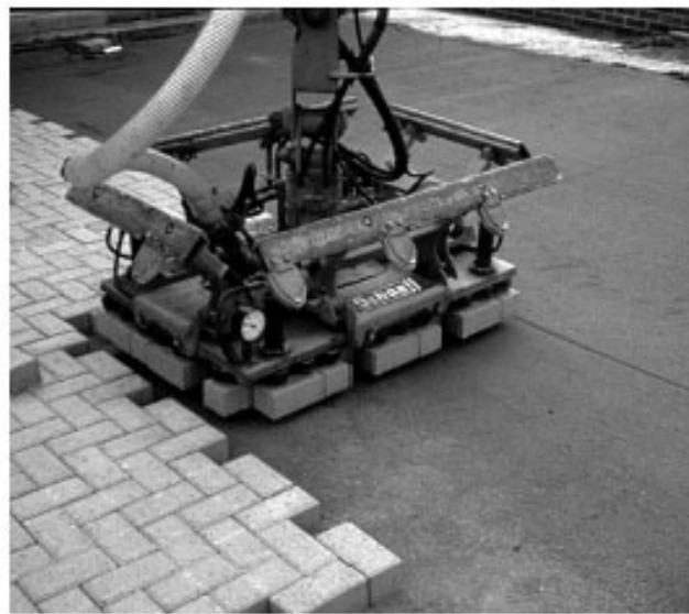
Figure 6. The vacuum head over the paver layer.
