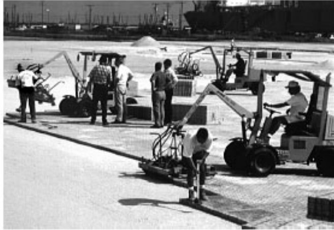
Figure 9. Mechanical installation equipment places concrete pavers rapidly.
