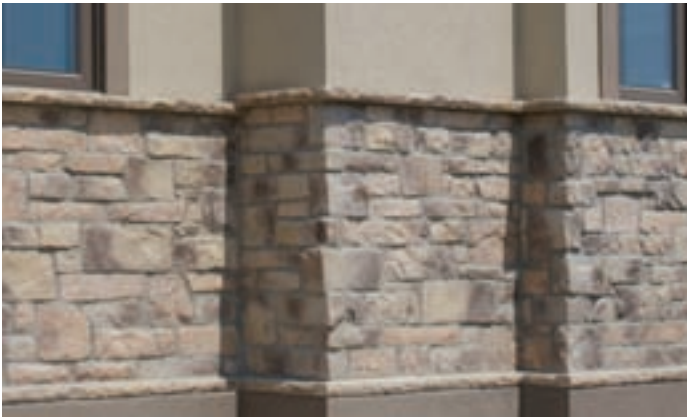
FOUNDATION SILL AND WINDOW BAND SIZES 24" X 3" X3"
