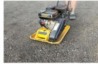
Next the 1/4" Washed Crushed Stone (HPB) is to be installed and levelled, keeping in mind to slope away from the building foundation and structures from the highest point to the lowest point. This will allow proper drainage and will prevent standing water
