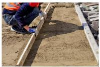
To install the stones carefully lay them into place and gently tamp them with a rubber mallet. Joint spacing can be left at your desired size. The stones can also be installed with no joint spacing as well.
