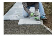
When all the stones are in place and levelled/sloped properly, the joints can be swept full with polymeric sand. Kindly follow the instructions of the polymeric sand manufacturer, keeping in mind to keep the sand within the joint. Polymers in the sand can stain the stone if left on the surface.
